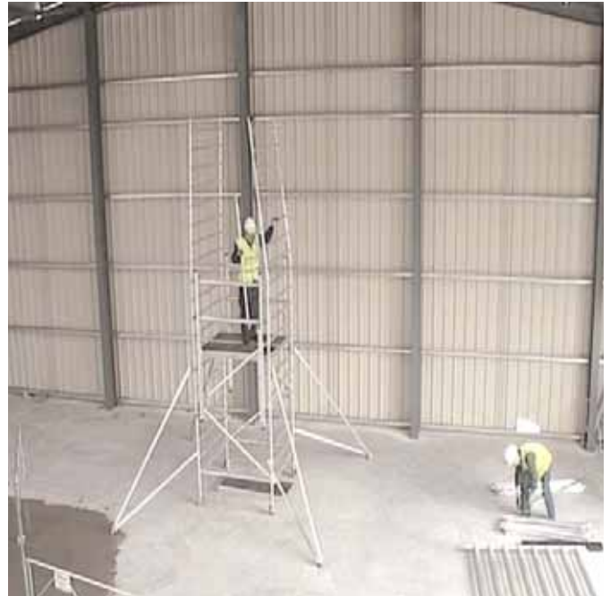
Figures 1 and 2 Advance guard rail
