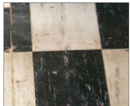
Asbestos paper linings can be found in boiler casings, under lino or tiles and many other places. Paper gaskets can contain asbestos
