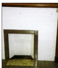
Asbestos insulating board (AIB) fire surround
