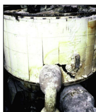
Asbestos lagging on an old tank
