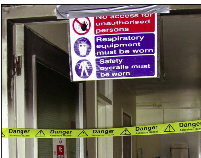
Make sure you restrict access
