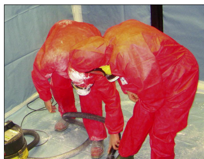
'Buddy' cleaning using a Class H vacuum cleaner
